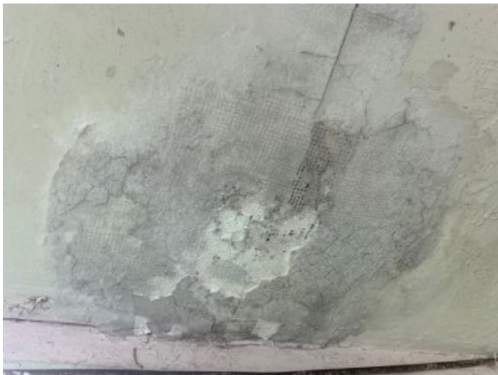
Eaves under front porch has been repaired with interior drywall compound.
